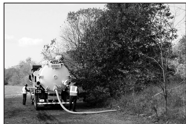
East Haven and New Haven associates work together to clear the grease-clogged line.
