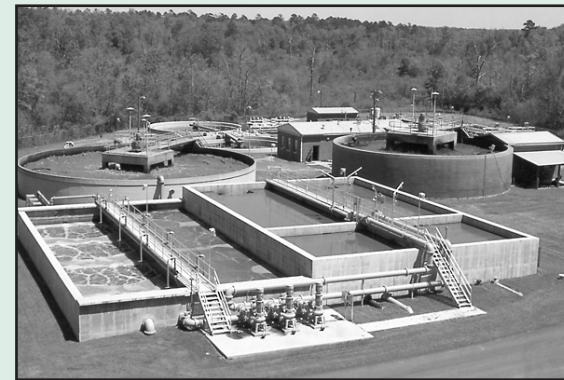
A view of the Quincy, Fla., plant.
