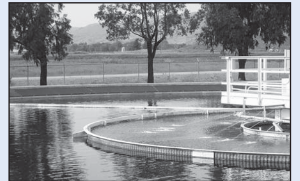
Covers added to the Gilroy/Morgan Hill secondary clarifier helped reduce the amount of algae growth and person hours needed to tend to the issue.
