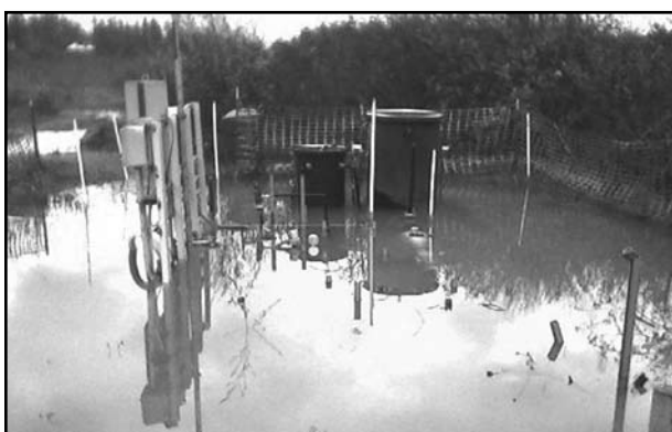
A view of the groundwater extraction well, where nearly 9 inches of rain caused flooding.
