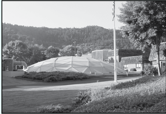
A view of the Roseburg, Ore., wastewater treatment plant.
