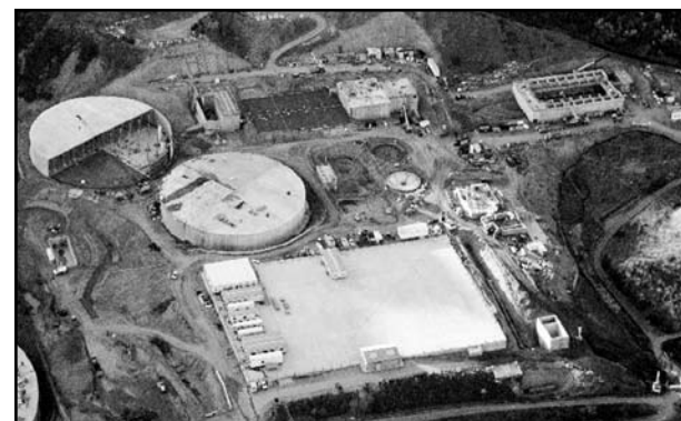
A view of the plant construction.
