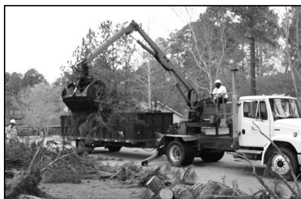
Associates help clear fallen trees after the tornado.
