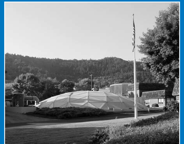
A view of Roseburg Urban Sanitary Authority's wastewater treatment plant.
