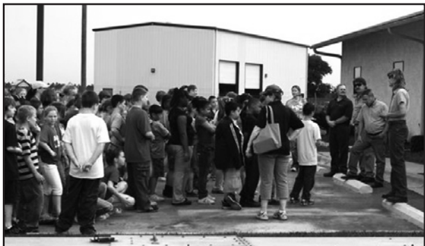
The Crestview team welcomes more than 100 fifth graders to the wastewater facility.
