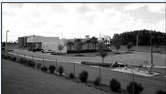
A view of the Ave Maria facility, which was designed and built by CH2M HILL. Our associates have operated the water and wastewater facilities since their inception. In addition to the Project of the Year Award mentioned in this article, CH2M HILL was awarded the national Merit Award from DBIA in November 2007.
