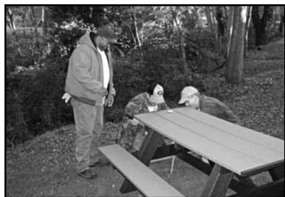
From left to right: Washington, Ga., Operator Darius Jenkins , Operator Greg Fanning and Sales Director George Cartledge secure a new picnic table they installed at Fort Washington.
