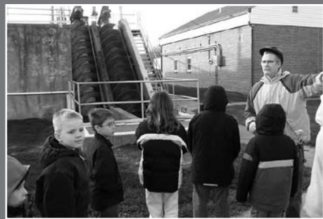
Associate Matt McAndrew , right, describes the direction of sewage flow to the students. In the background are screw pumps, which elevate water after it's cleaned in grit chambers.
