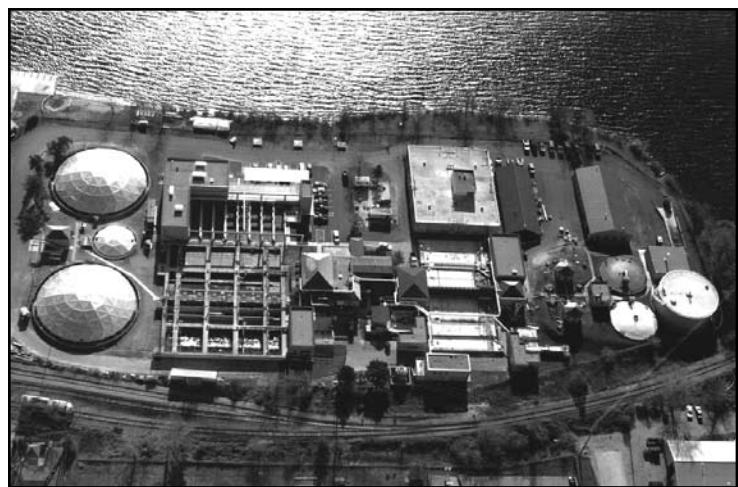
A view of the Traverse City plant.
